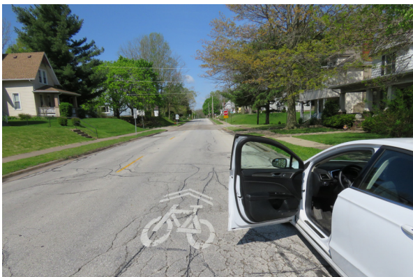
Figure 6.3 – Shared-Lane Marking Located Outside of the “Door Zone”
