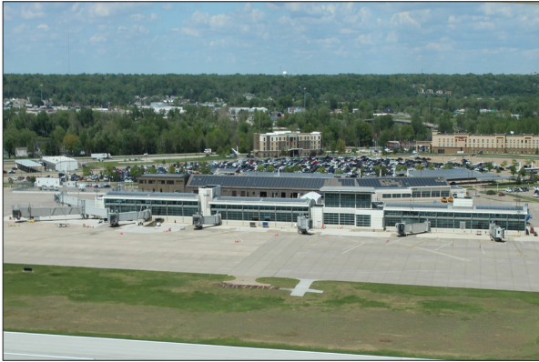
Source: Quad Cities International Airport
