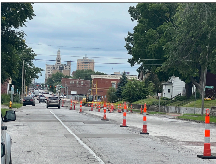
Figure 4.6 – Sample Road Construction, Davenport, Iowa
