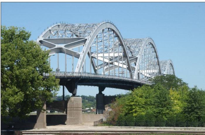
Figure 4.4 – U.S. 67 Centennial Bridge at Mississippi River, Rock Island, Illinois
