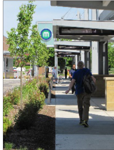
Figure 4.7 – MetroLINK District Station, Rock Island
