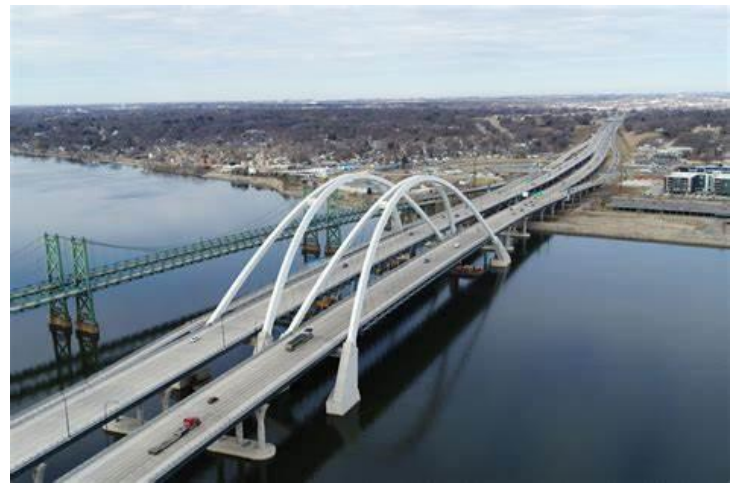
Figure 26: The Newly Constructed I-74 Mississippi River Bridge
