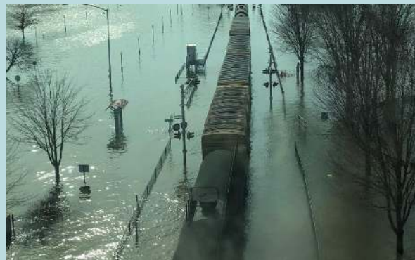
Figure 80: Flooded CP Track in Davenport
